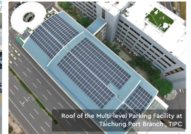
Roof of the Second Office of Taichung Port Branch, TIPC
